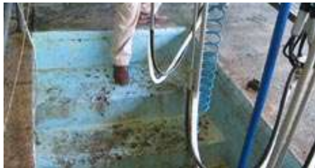
Figure 5. Concrete pit steps with generous tread dimensions are good for gumboots.
