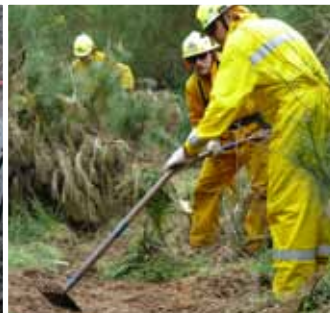
Middle: fire break construction using hand tools
