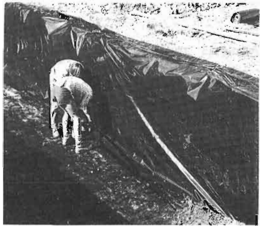
FIG. 2 (below)—Root-trench showing overlap and cementing of polythene sides to "Sarlon" mesh lining on bottom.
