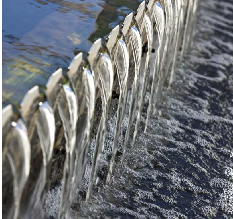
We help industry clients develop long-term solutions for improving wastewater treatment systems.
