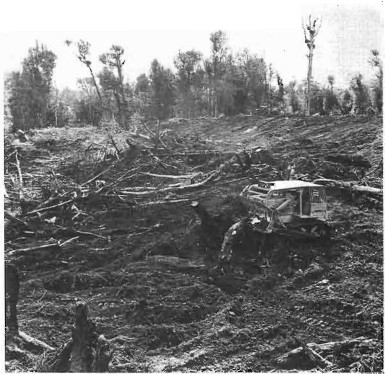
FIG. 4—Bulldozer clearing indigenous cutover bush for establishment of P. radiata . Such stump and root removal should substantially reduce the normally high losses to Armillaria root rot that are characteristics of P. radiata established on certain indigenous cutover sites cleared by felling and burning without further site disturbance.
