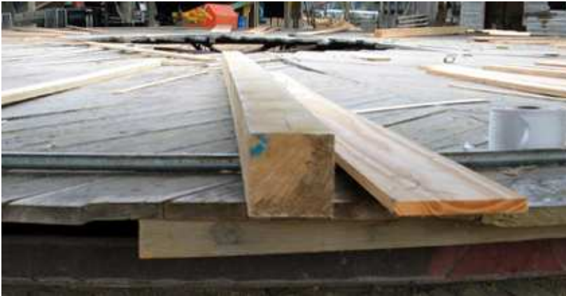
Pipe fitted on green table edge to reduce friction
