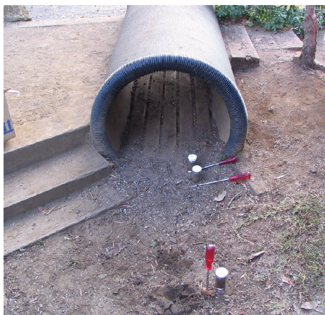
Figure 2. Queens Park, tunnel with decking floor installed in 1998.
