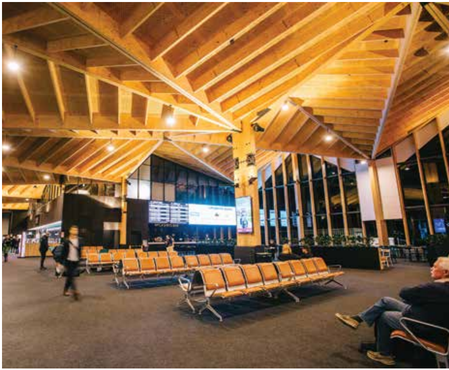
The recently opened Nelson Airport terminal is a great example of a new timber construction with engineered wood products that are storing carbon long-term.
