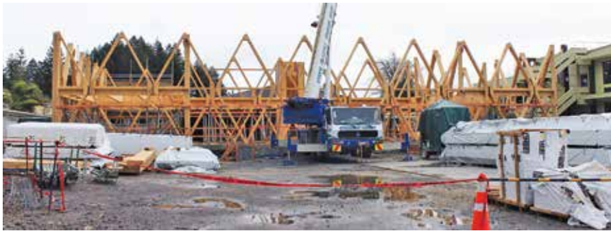
Progress is quick on Scion's Innovation Hub. Photo taken on 21 August.
