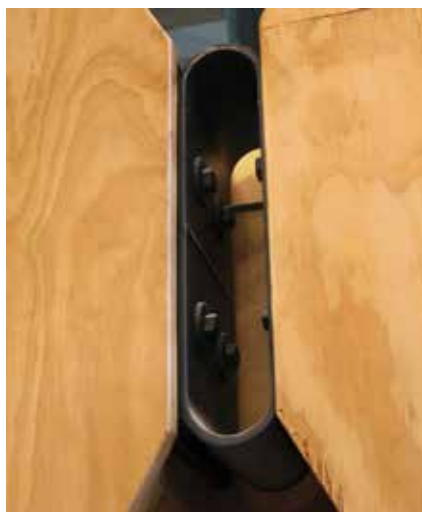
UFP plates absorb and disperse seismic energy.
