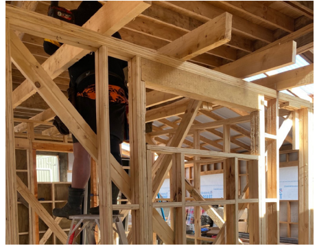
Roof and wall frames.
